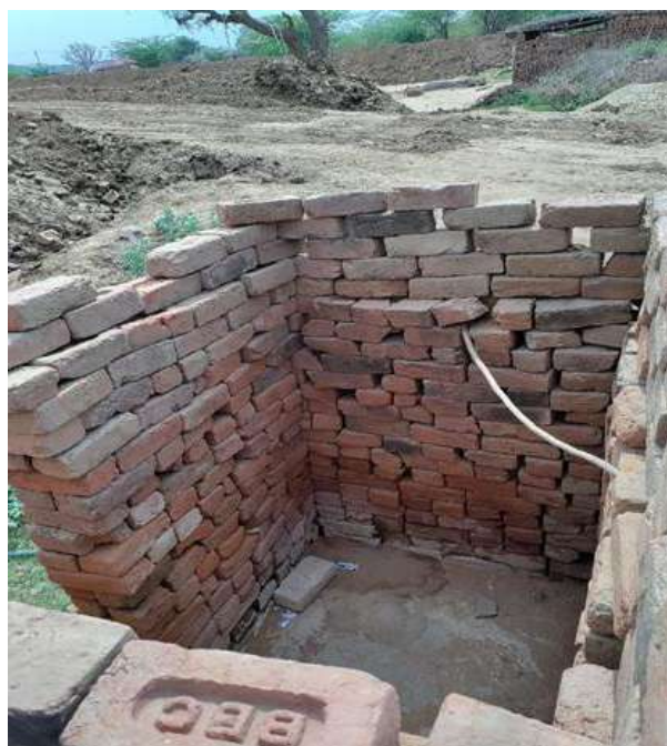
Self-constructed temporary bathroom structure for the use of women workers in BBC Ladpura (Ajmer)
